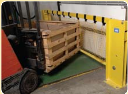
Reduce damage to doors and door tracks
